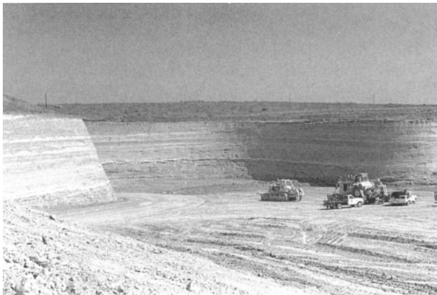
Fig. 14.1.4.3. Stripping operations—overburden removed and rock exposed for drilling.
