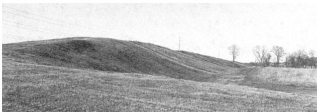
Fig. 14.1.7.1. View of boundary berm construction.
