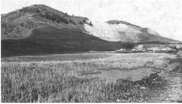
Fig. 14.1.5.1. North Henry mine area showing backfilled pit in the center (dark area). Aerial photo.
