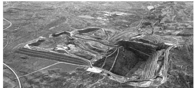
Fig. 14.1.6.1. Aerial photograph of the Kemmerer mine (1-UD pit) looking south.
