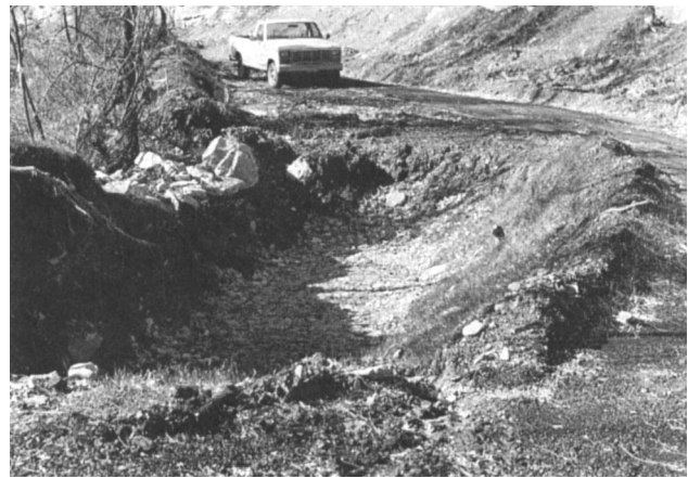
Fig. 14.4.1.1. Typical sediment control structure on an auger bench.
