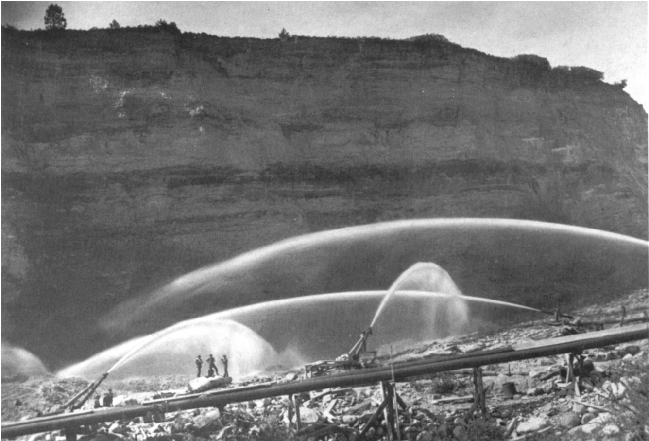
Fig. 22.3.1. Early water-jet monitor being used in Idaho (Idaho Historical Society).
