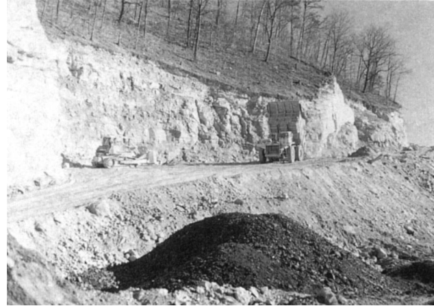
Fig. 14.3.5.7. Final highwall slope configuration.
