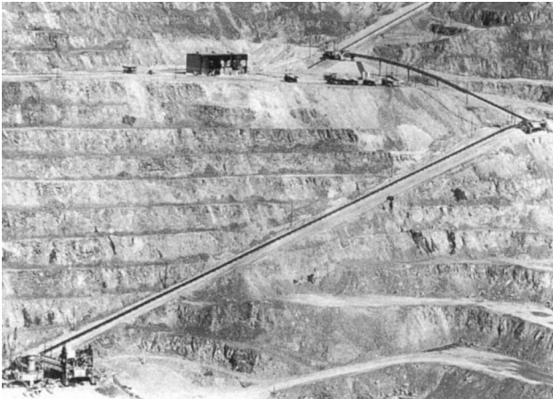
Fig. 13.5.8. Conveyor flights leaving a pit via switchbacks.
