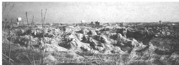
Fig. 14.1.7.2. Preparation of top bench.
