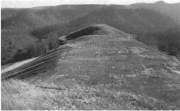
Fig. 14.3.5.8. Reclaimed mountaintop removal area.
