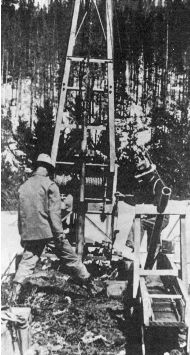
Fig. 5.3.12. Airplane placer drill (Wells, 1969, p. 51).
