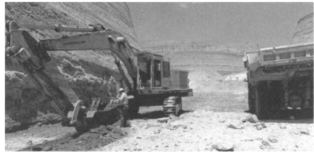
Fig. 14.1.4.4. Probing material in backhoe bucket for grade control.
