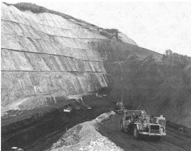
Fig. 14.1.5.2. General pit workings, 1989.
