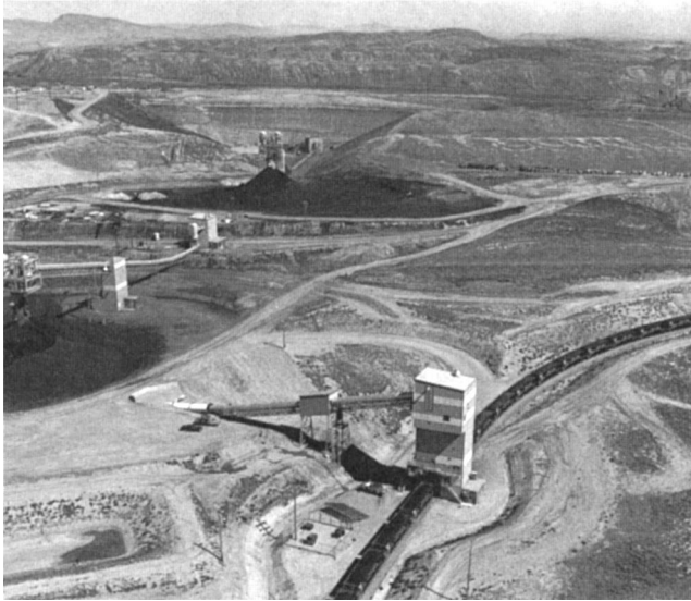
Fig. 25.2.24. Unit train loading facility. Storage bin fed by sloping conveyor stores sufficient coal for continuous loading of 100-car unit train with 100 tons (91 t) per car. (courtesy: A.T. Yu).
