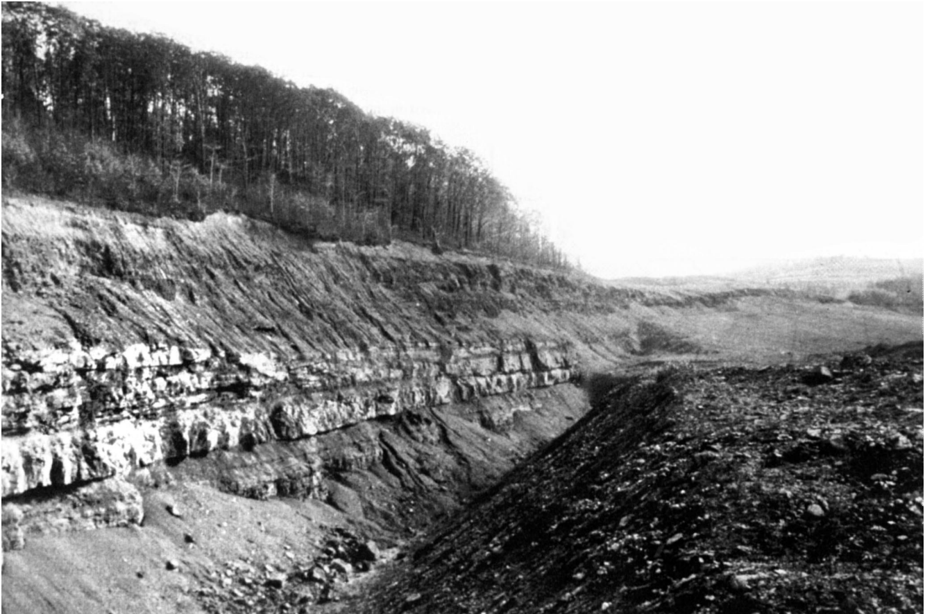
Fig. 3.4.1.2. Unreclaimed strip mines pose environmental and public safety hazards.
