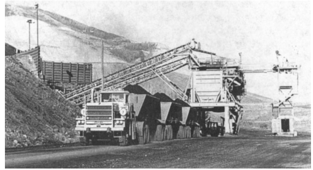
Fig. 14.1.5.7. Henry tippie and ore transport truck and trailers.
