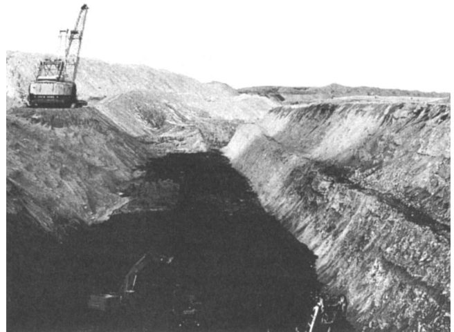
Fig. 14.3.1.6. Dragline on the spoil side.
