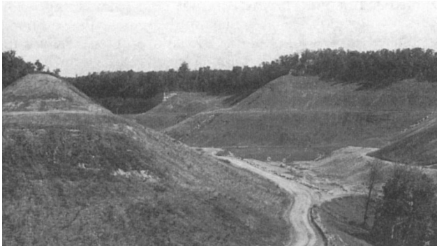
Fig. 14.3.5.5. Typical mining area.
