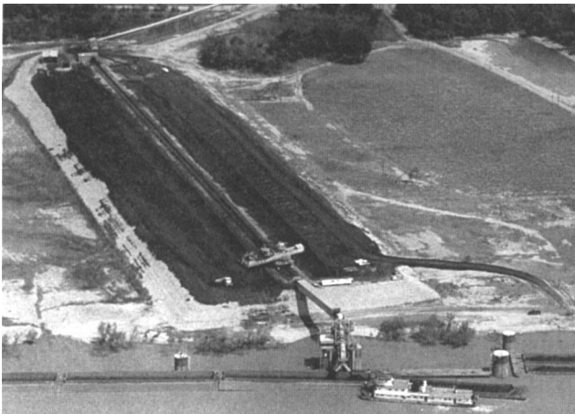
Fig. 25.2.14. Ten-mile (16-km) long cable belt overland conveyor from mine to open storage. Bucket wheel stacker-reclaimer supplies barge loading river dock (courtesy: McNally-Wellman).
