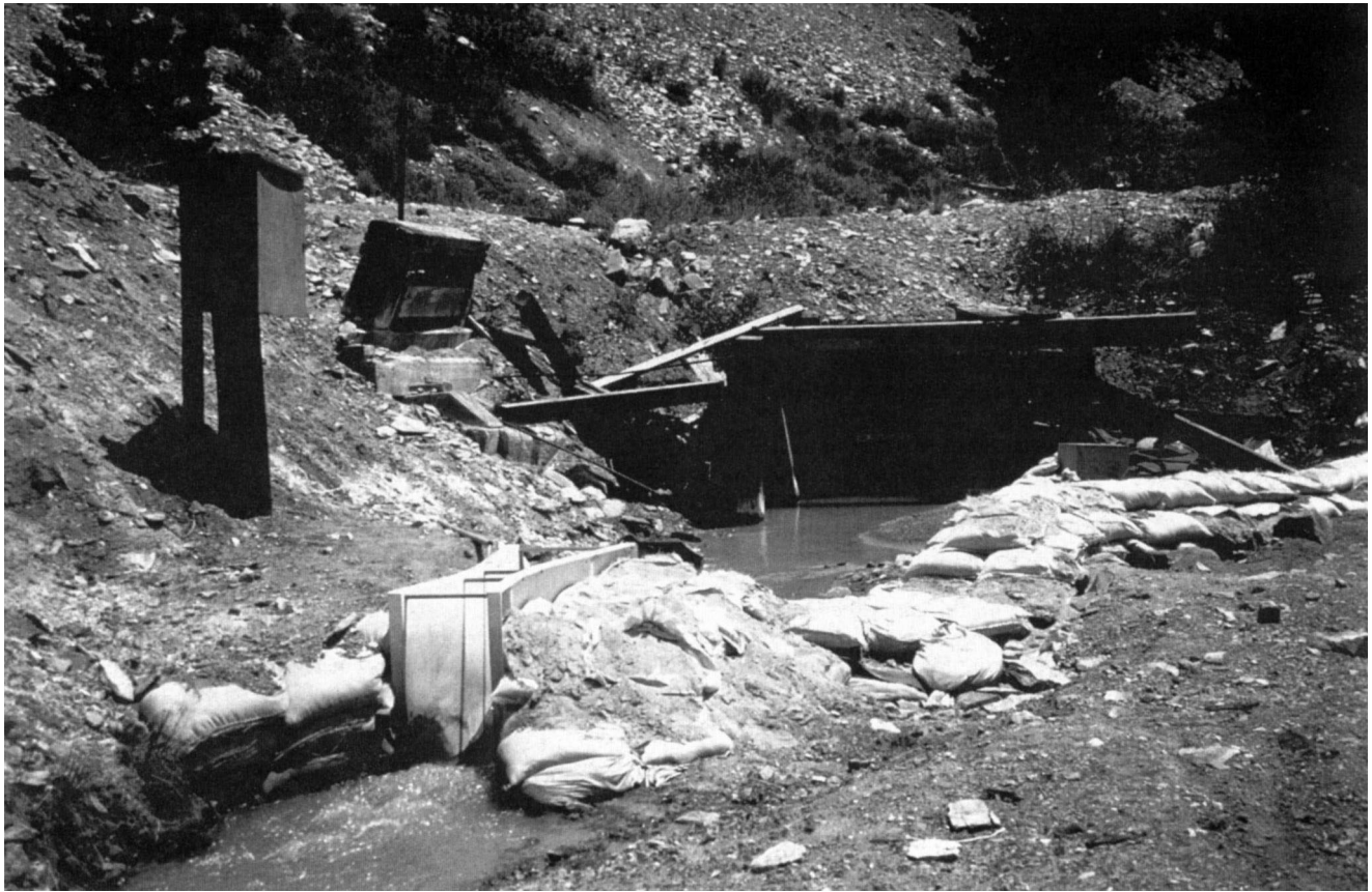
Fig. 3.4.1.4. The Yak Tunnel, part of the California Gulch Superfund Site, drains acid, metal-laden water from the Leadville, CO, mining district.
