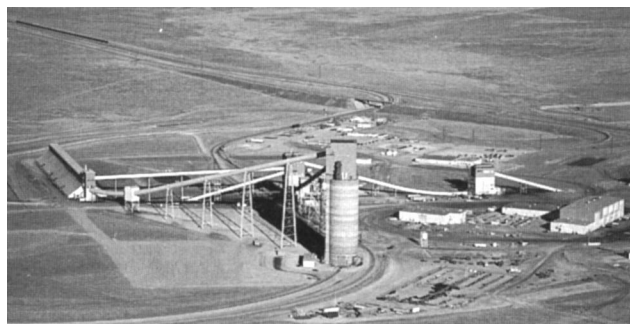
Fig. 25.2.8. Covered storage complex with rectangular covered roof at left for long-term storage. This feeds the concrete silo in center foreground. Unit train will pass under silo for flood loading (courtesy: PEBCO).
