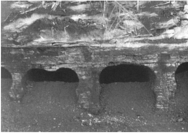
Fig. 14.4.1.3. Hole configuration and remnant web.
