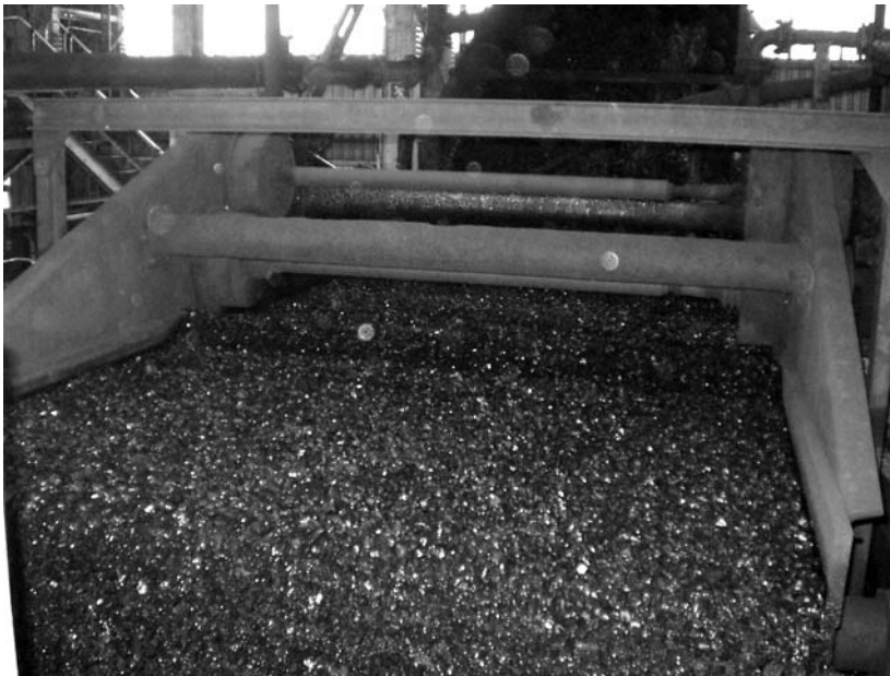
Fig. 1.1.1 - Screening at Anglo Coal's Kleinkopje coal preparation plant, South-Africa [TU Delft].
