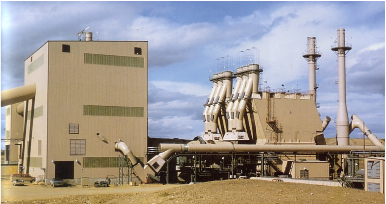
Coal drying plant [KHD Humboldt-Wedag]
