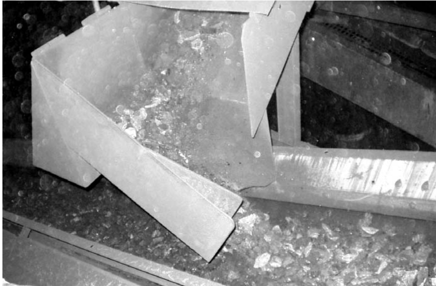
Fig. 6.1 - Dust generation at a conveyor transfer point.
