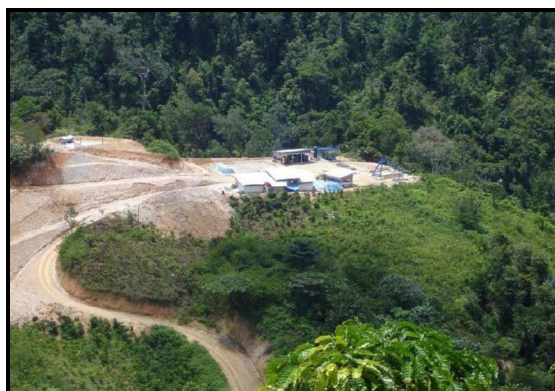
The modern Way Linggo mine on Sumatra (2010)
