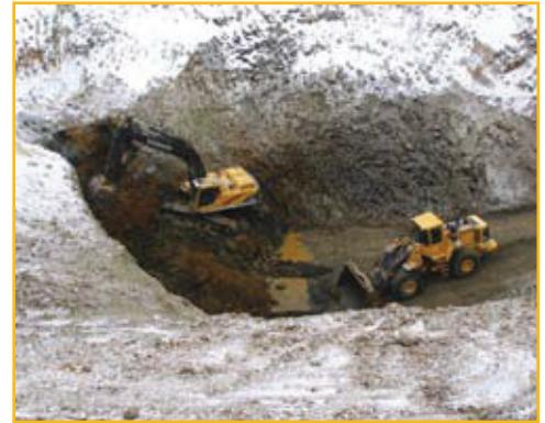
Portal preparations for the bulk sample drift at Stora Sahavaraa, Sweden.
