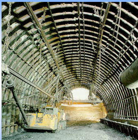
Steel support with boarding
