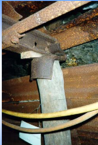
Frame support with wood and steel
