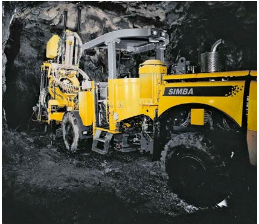
Longhole drilling with Simba M4 C in the Burkland stopes.
