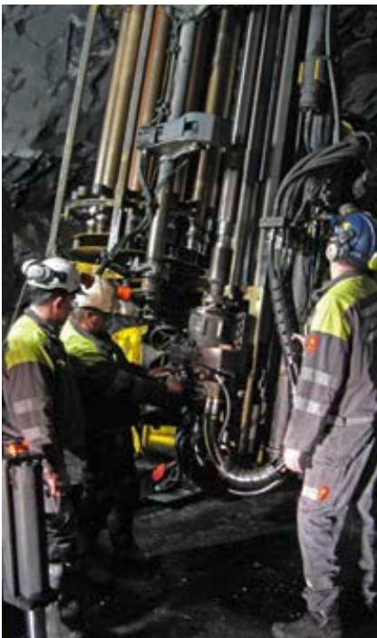
Setting up a Simba W6 C for production drilling.
