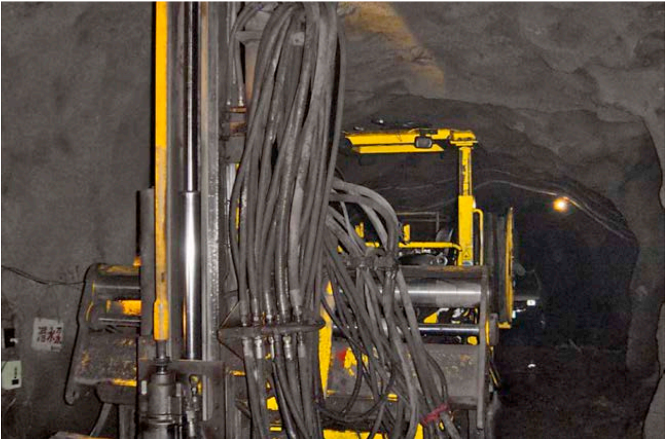
Simba production drill rig, one of six at Meishan.
