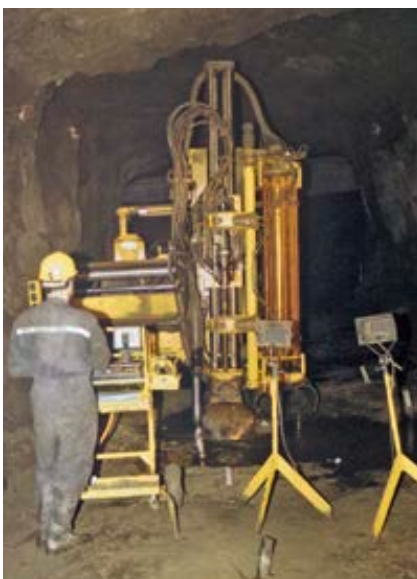
Production drilling with Simba H1254.
