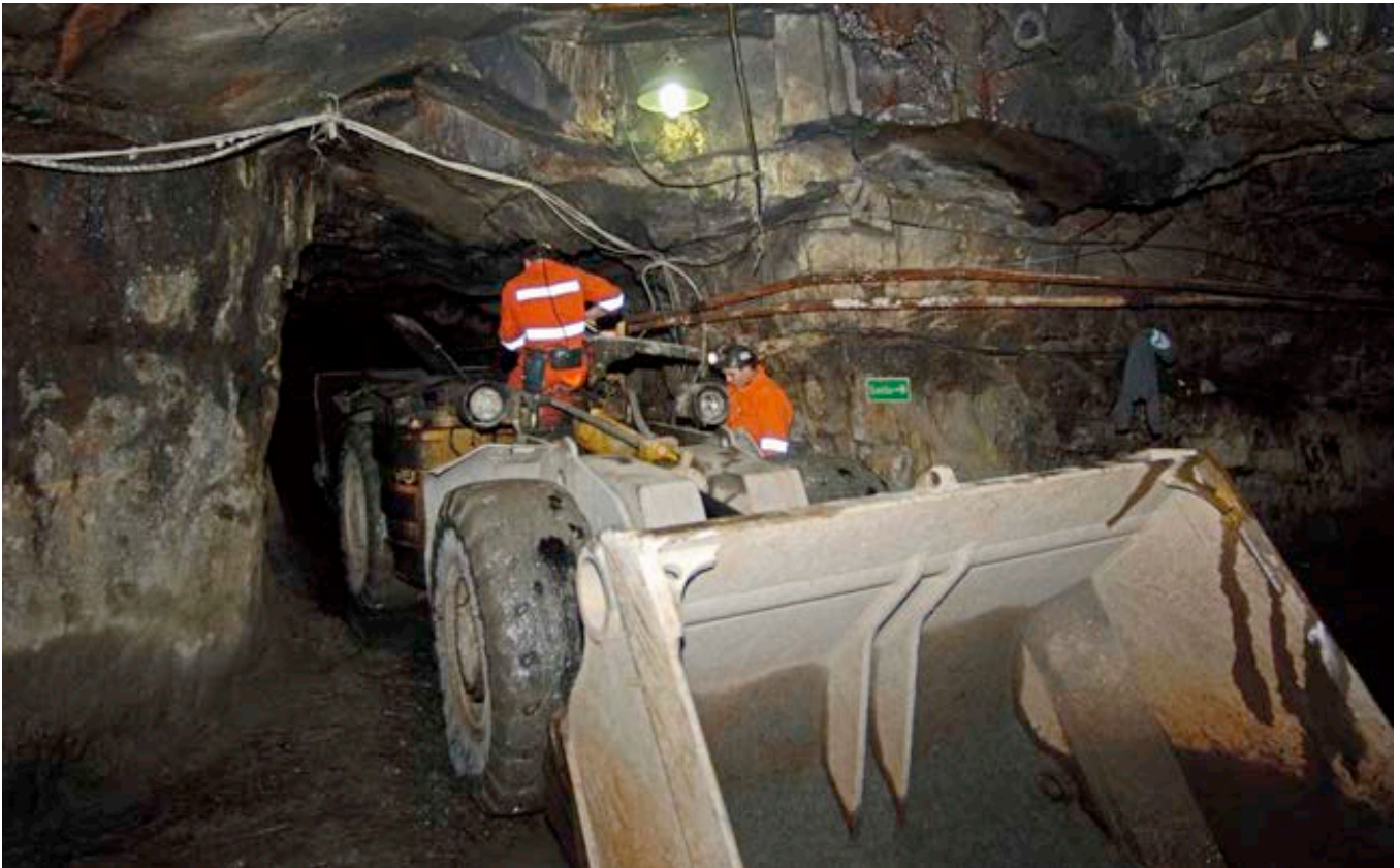
Scooptram ST600LP under maintenance.
