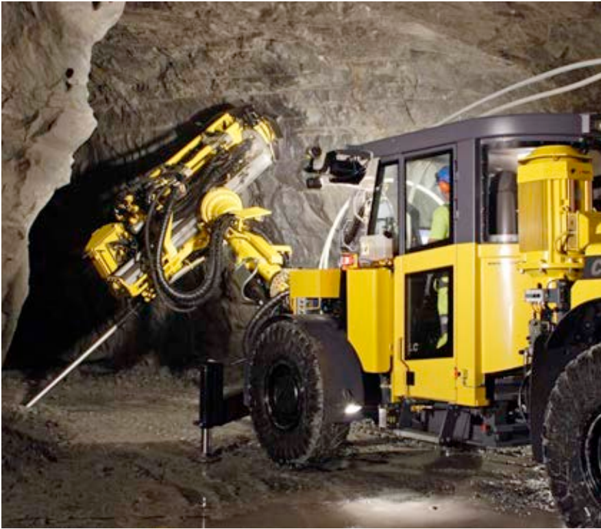
Mechanized cablebolting with Cabletec LC.
