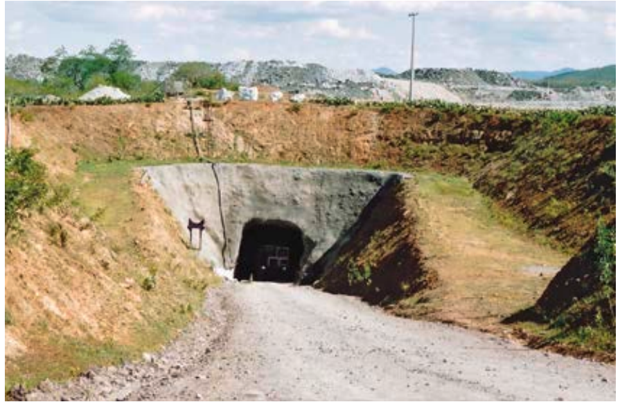
Entrance to the Ipueira mine.
