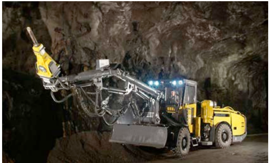
Mechanized scaling with hydraulic hammer.
