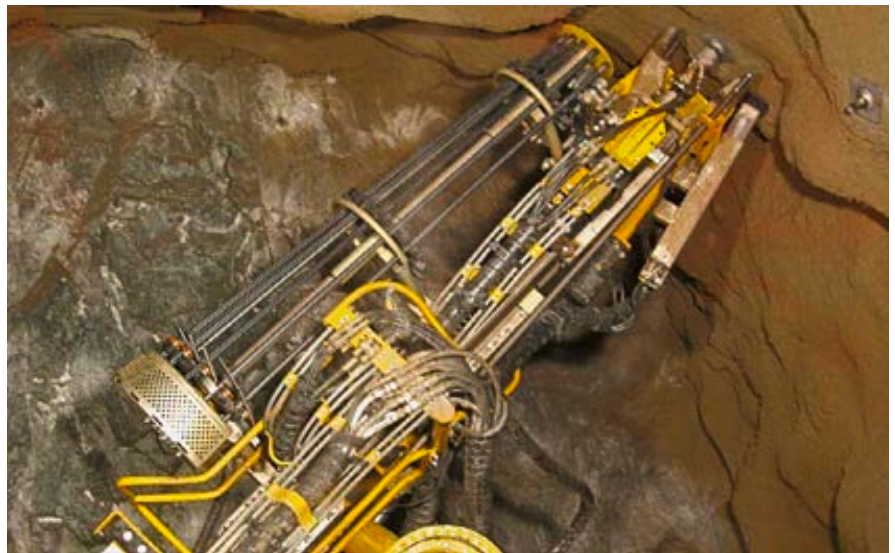
Boltec LC installing Swellex Mn12 rockbolts.
