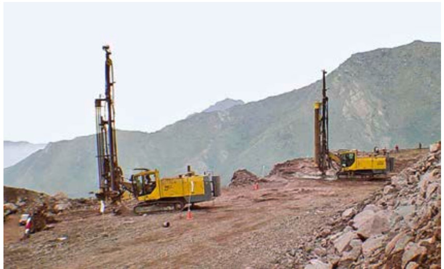
Atlas Copco ROC L8 crawlers at El Soldado open pit.
