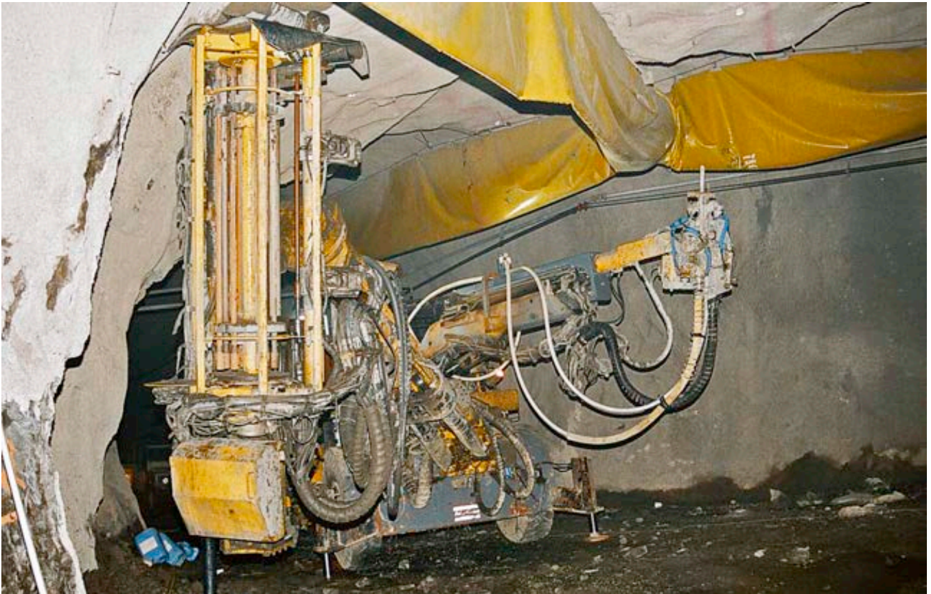
The mine's Cabletec in action.
