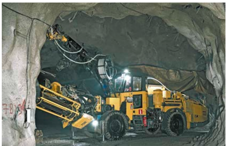
Cabletec L installing cable bolts at Kemi.
