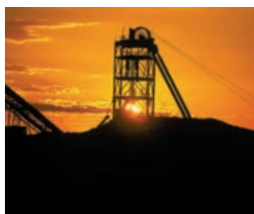
Front cover: Headframe at Australia's Golden Grove mine.
