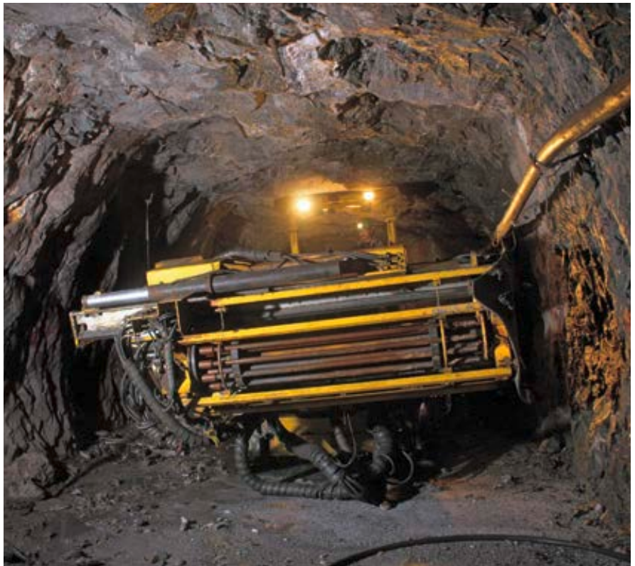
Setting up Simba 1254 for blast hole drilling.
