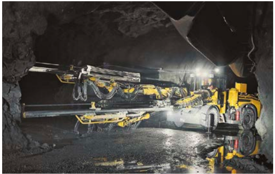
Rocket Boomer L2 C is used for sublevel development.
