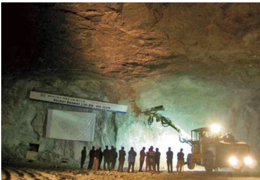
Rocket Boomer L1 C-DH on demonstration at Yongjeung limestone mine.
