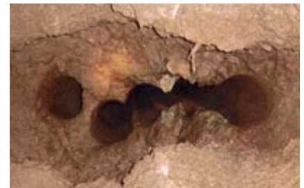
Holes at breakthrough after 32 m.
