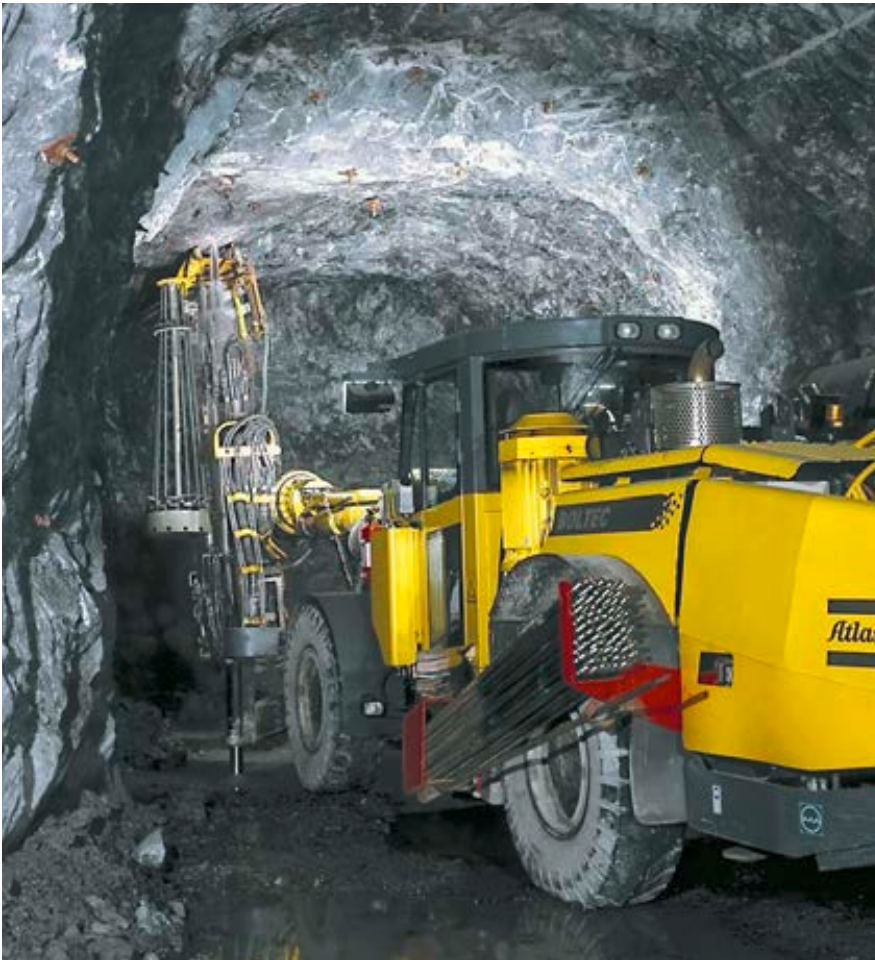
Boltec LC installing rockbolts in a development drift.
