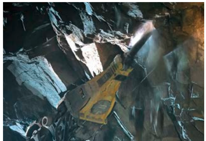
Close-up of the Scaletec at work.
