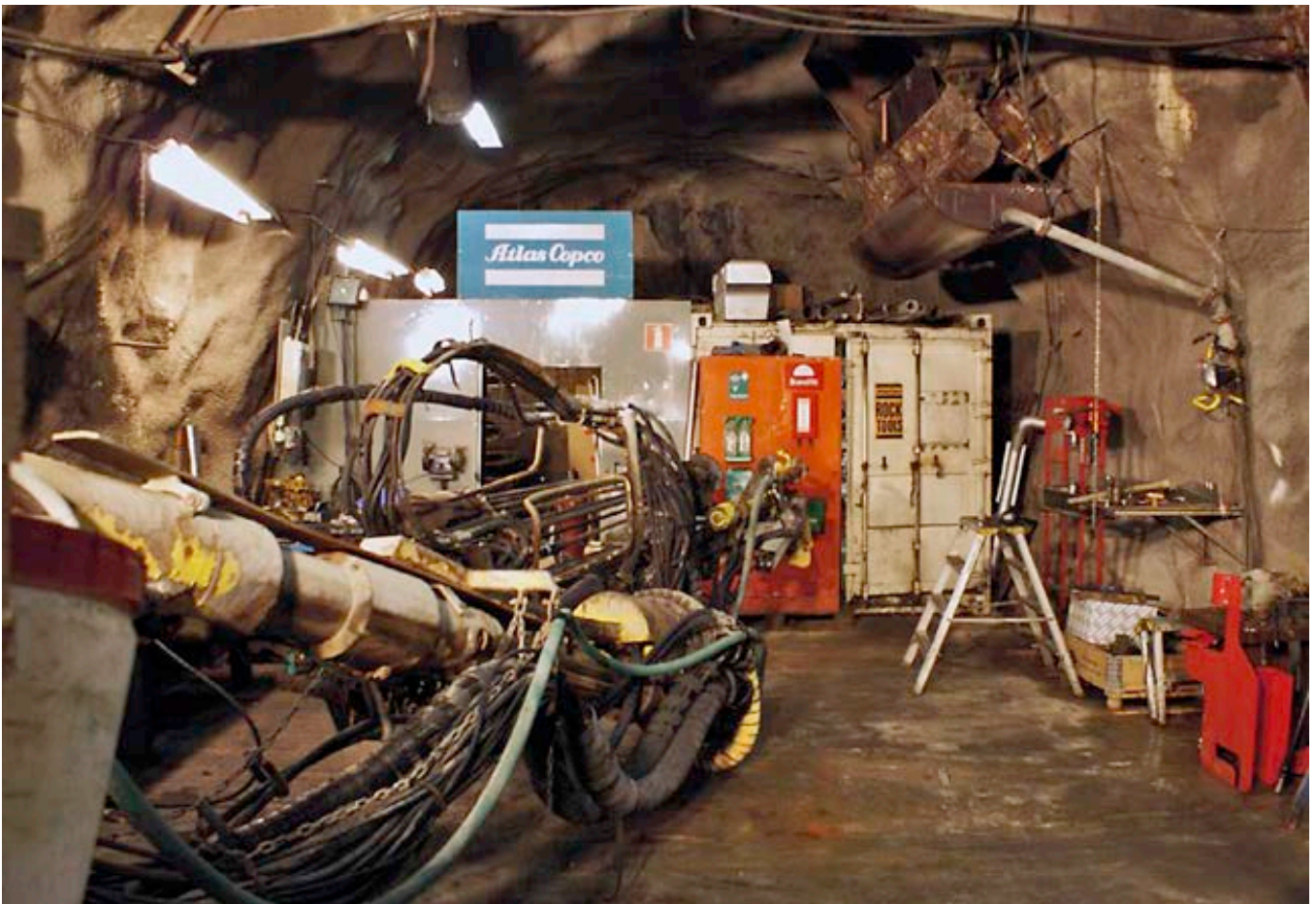
Boltec LC in for service.
