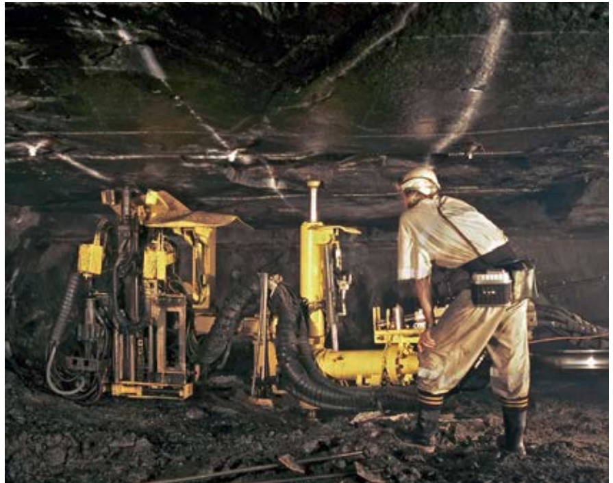
Roof bolting in low headroom.
