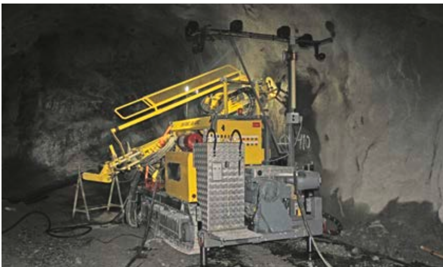
Atlas Copco Diamec U6 APC at work underground.
