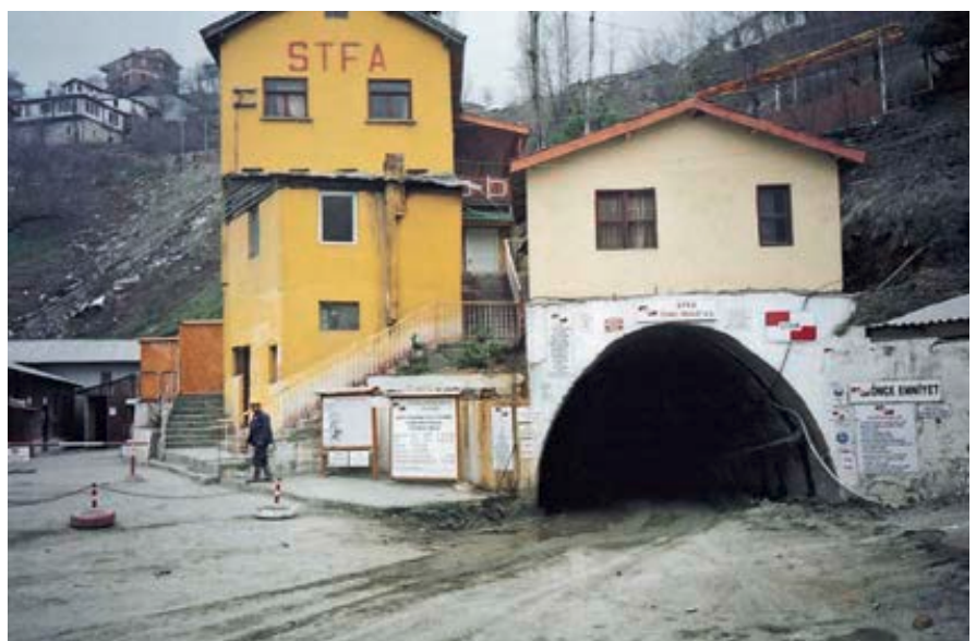
Portal entrance to Asikoy underground mine.
