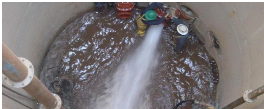
Figure 4.18 Looking down into the large caisson of a horizontal collector well, with water discharging out of one horizontal collector well. Note the two men at the bottom for scale (photo courtesy of Layne Christiansen Company).
