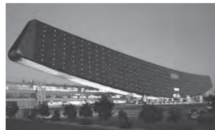
FIGURE 37.20 Japan's Sanyo Solar Ark incorporates some 5000 photovoltaic panels and generates a peak power of 630 kW.
