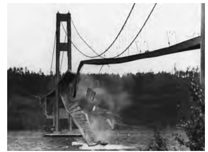
FIGURE 13.26 Collapse of the Tacoma Narrows Bridge—only four months after its opening in 1940—followed the resonant growth of large-amplitude oscillations.
