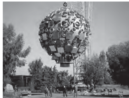
FIGURE 23.18 The NIF target chamber, shown during installation (Passage Problems 75–78)
